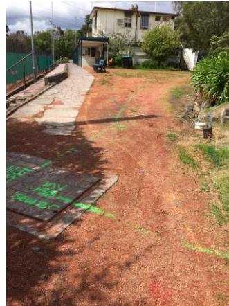
Service Detection markings
