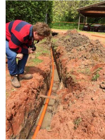
Robin inspecting the trench
