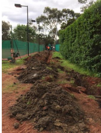
Trenching for the new cables
