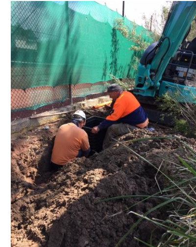
Placing the junction boxes
