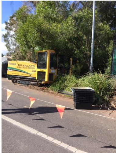
The drilling machine at work
