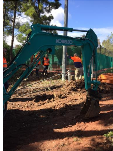
Pulling the conduit through the drilled hole
