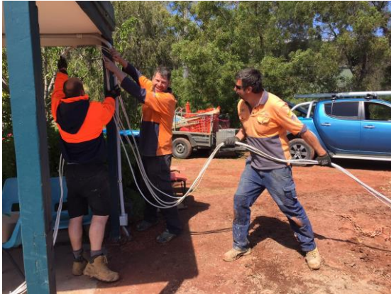
Laying the cables
