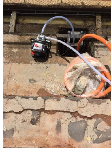
Footing hole outside clubhouse (waiting for concrete)
