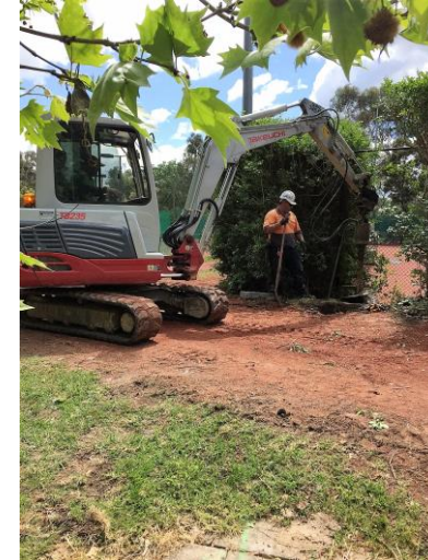
Digging the last pole hole at Court 6
