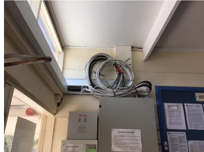
Cables ready and waiting to be attached
