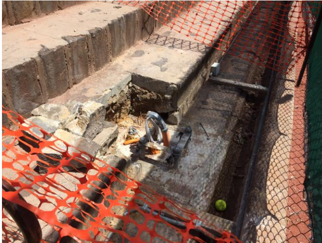
Footings & cables ready for the Pole
